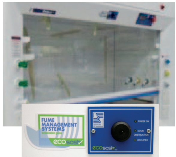
The EcoSash® Motion Sensor module is mounted on the face of the fume cupboard in the centre above the sash. Shown here on an Advanced Air® EcoAir® fume cupboard, the sensor panel can be easily mounted on any make of fume cupboard. It continually monitors operator activity and communicates with the EcoSash® Controller.
